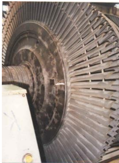
Figure 2 Blades of end stage.
